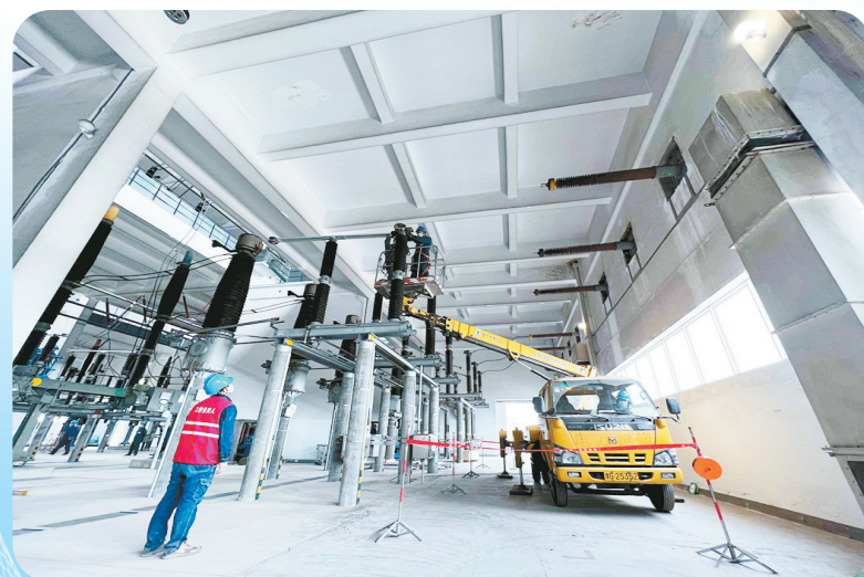
变电站安装刀闸
